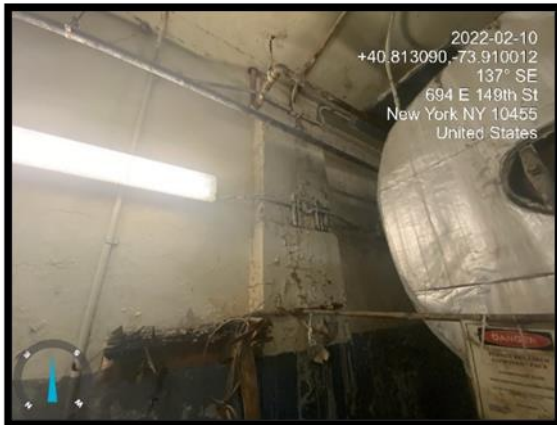
Photo 14. Current Wall Finish Conditions
