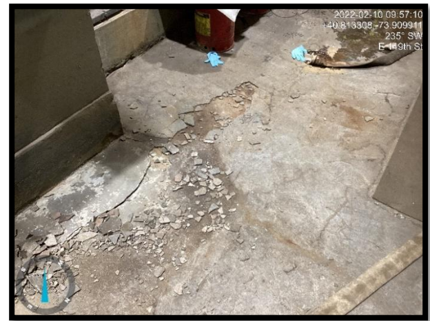
Photo 13. Current Floor Finish Conditions
