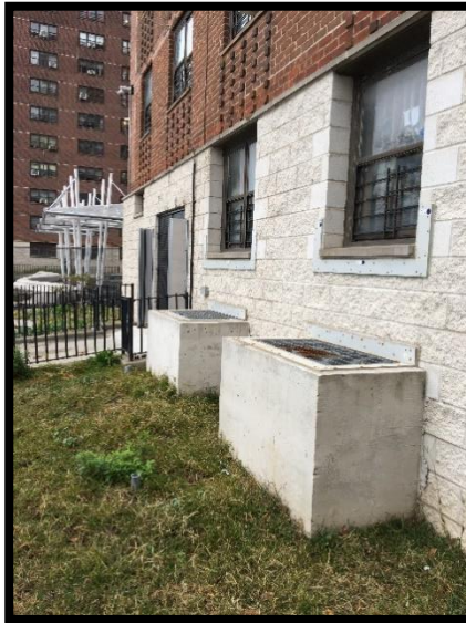
Photo 34. Flood Protection of Areaways
