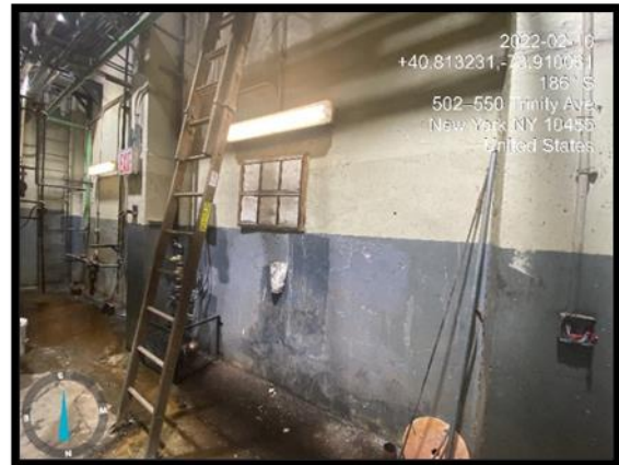
Photo 15. Current Wall Finish Conditions
