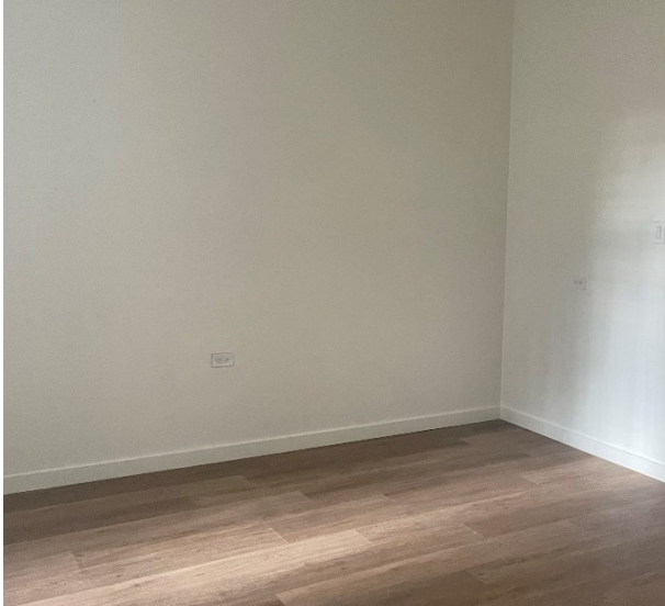
Frederick Samuel Apartments: Wood wall base
