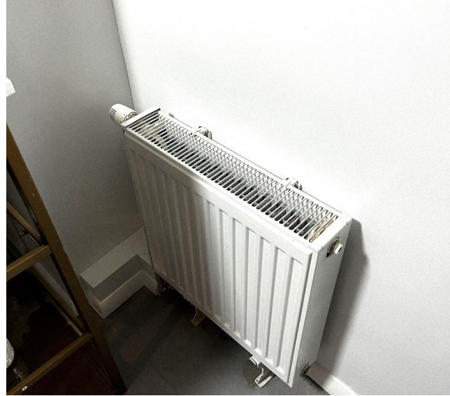
Williamsburg: New radiator covers and enclosed piping
