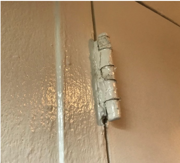
Existing conditions: painted door hinges
