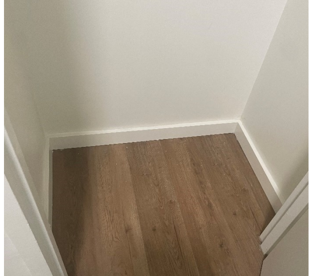
Frederick Samuel Apartments: Wood wall base in closet
