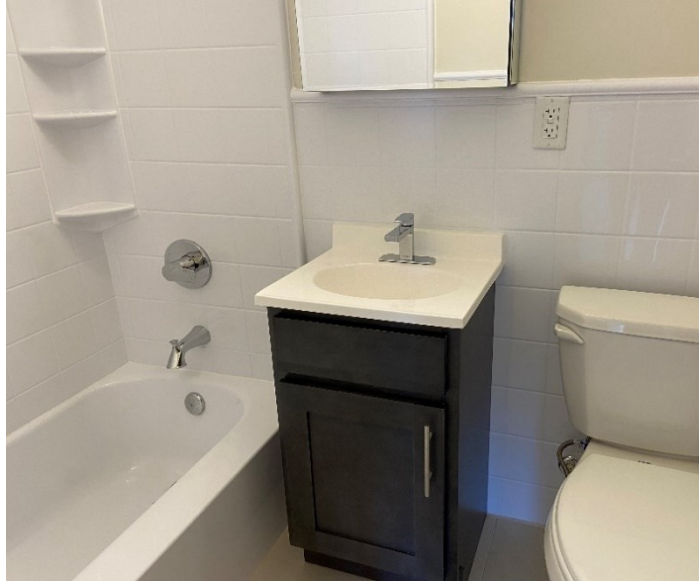
West Brighton: Vanity, tub, full height tiling
