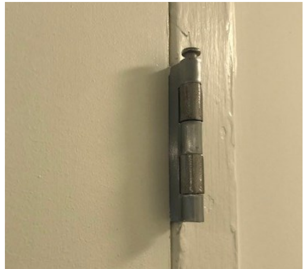
Jackie Robinson & Harlem Scattered Sites: existing hinges with stripped paint and rewelded to frame and new door
