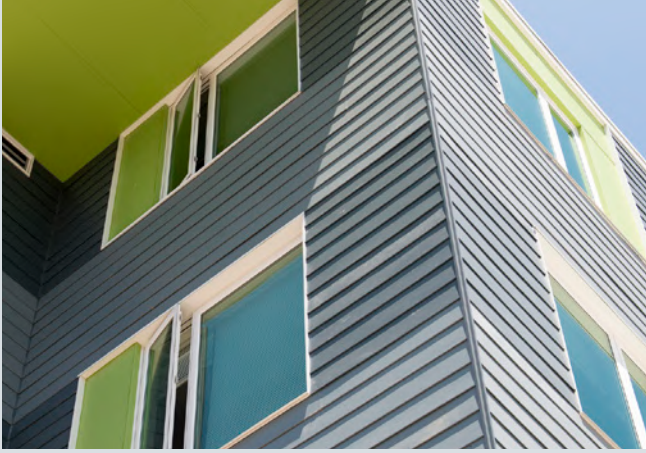
uPVC casement windows tested and used in a supportive housing in Madison, WI Photo: Heartland Housing
