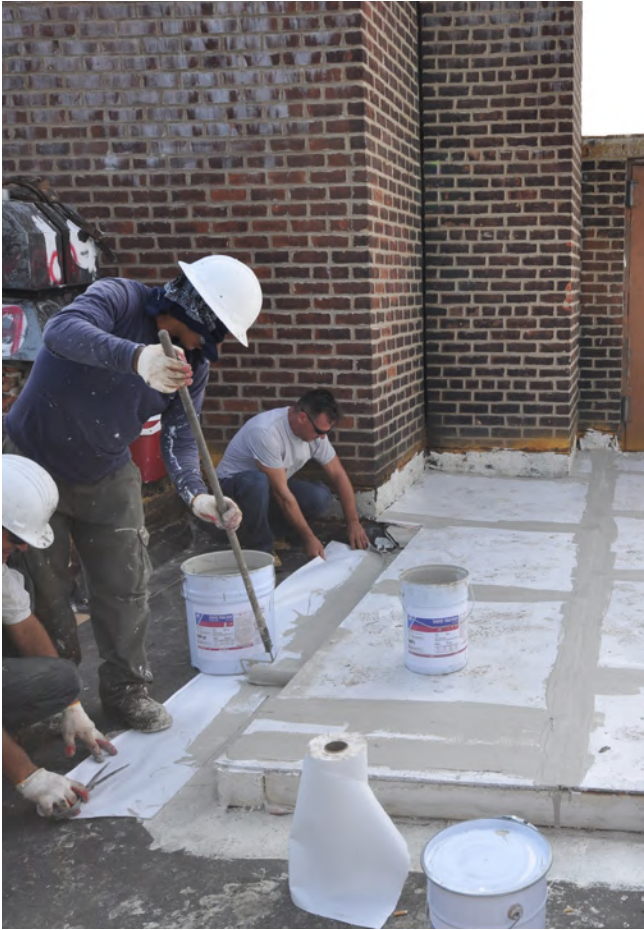
Roof insulation installation Photo Tom Sahagian
