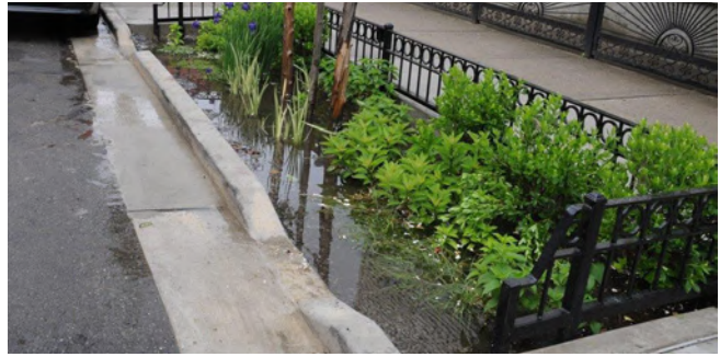
Right-of-way bioswales and stormwater greenstreets are planted areas in a sidewalk or roadbed that capture curb runoff. They are installed over a layer of broken stone with engineered soil and topped with appropriate plants and trees.
