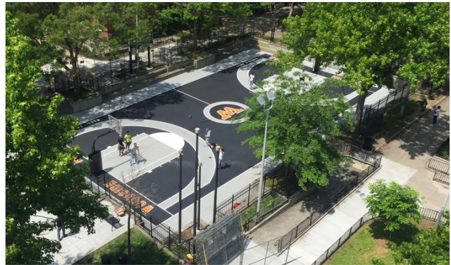
Basketball court rehabilitation at Woodside Houses
