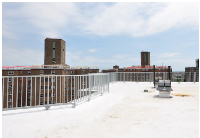
Completed roof rehabilitation.
