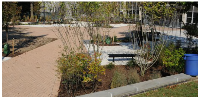
Porous paving can be configured to either allow water to infiltrate through the paver joints or through the paving itself. As with the other systems described above, porous paving is installed over a base of broken stone (see more next page).
