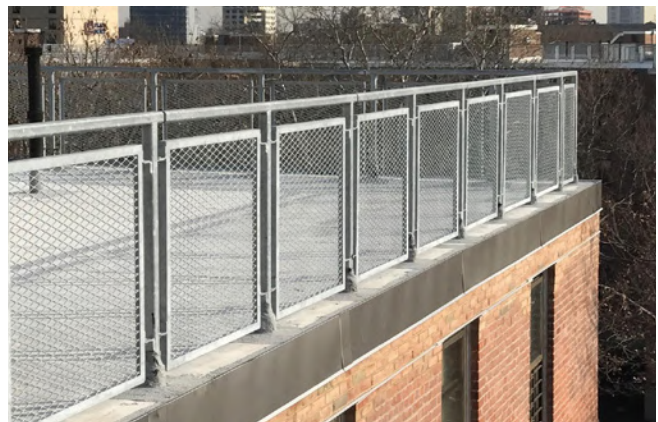
Rehabilitated parapet walls
