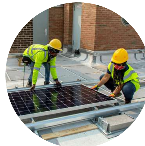
Solar panel being installed at Queensbridge Houses.
