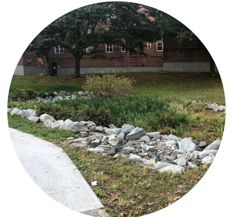
Green infrastructure installation at Edenwald Houses.
