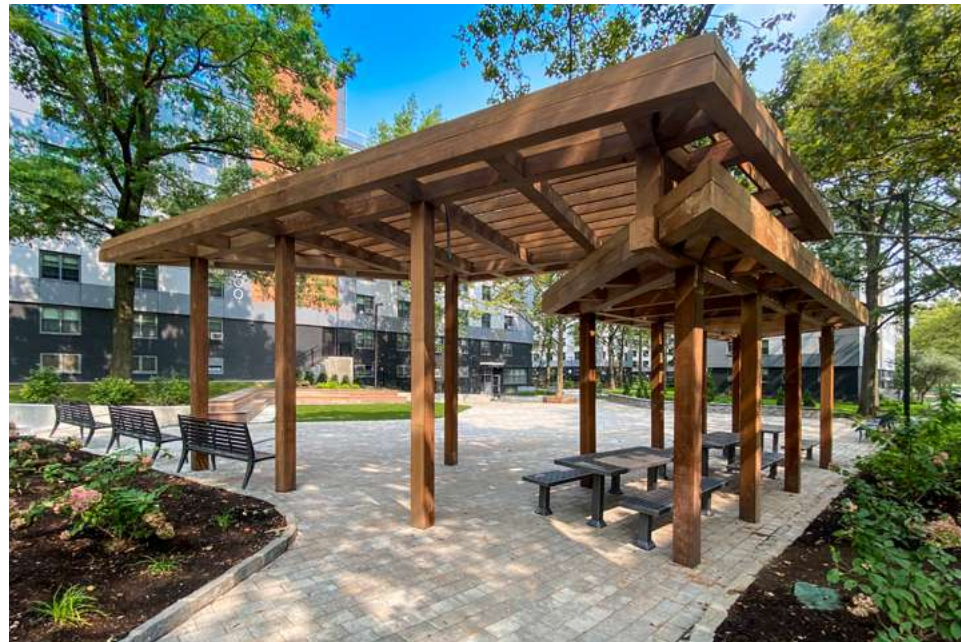
Renovated court yard at PACT development, Baychester. © Andy Foster
