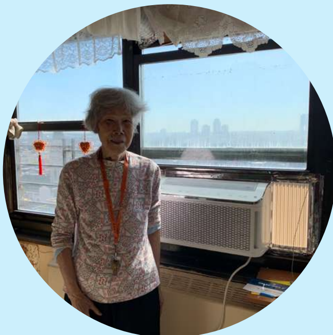
Resident standing next to newly installed "smart" AC at Meltzer Towers.
