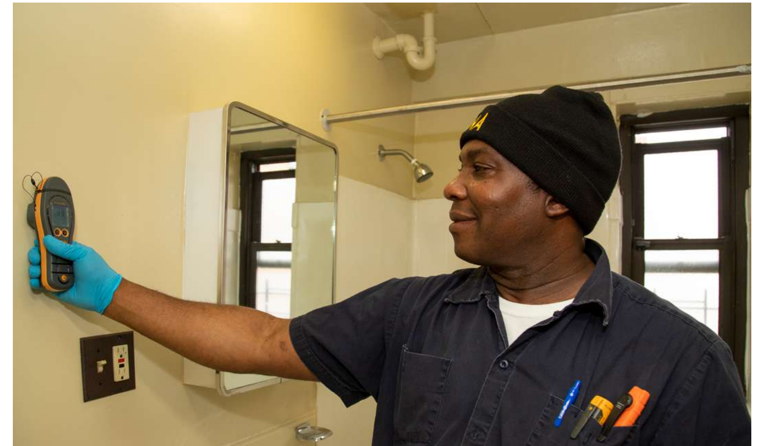
The Mold Busters process introduced new mold inspection tools including the Protimeter, a surface moisture detector.
