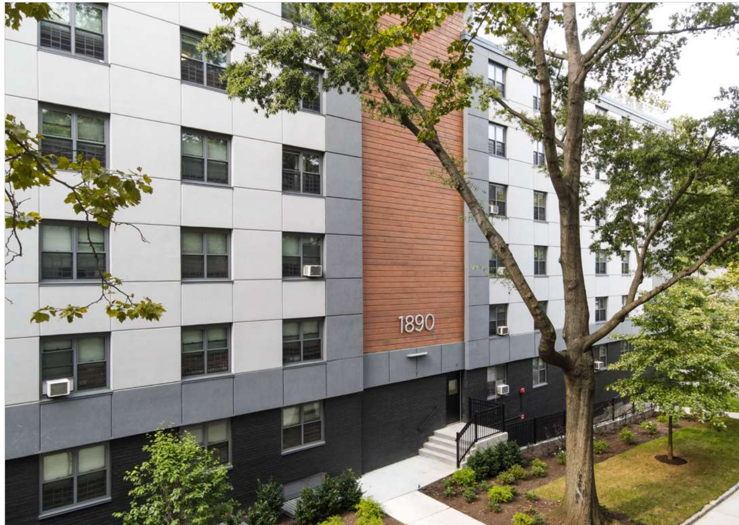
Renovated façade at converted PACT development, Baychester Houses ©Andy Foster
