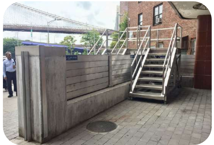
The deployable stairs in Smith houses can be bolted to the ground for stability
