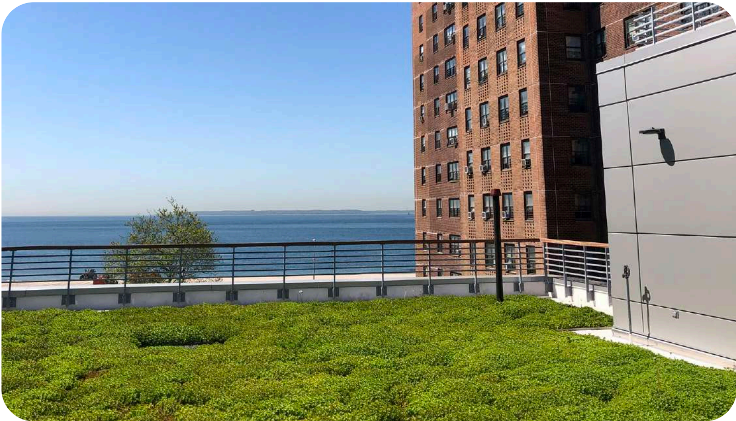
Green roof on top of the boiler plant at Coney Island Houses
