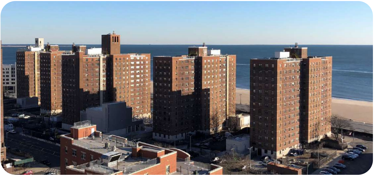
Rooftop generators at Coney Island Houses
