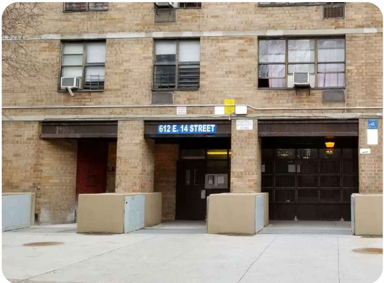
Passive barriers at Campos Plaza
