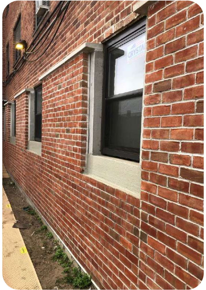
Gravesend: Structural reinforcement was designed to blend with the existing facade.
