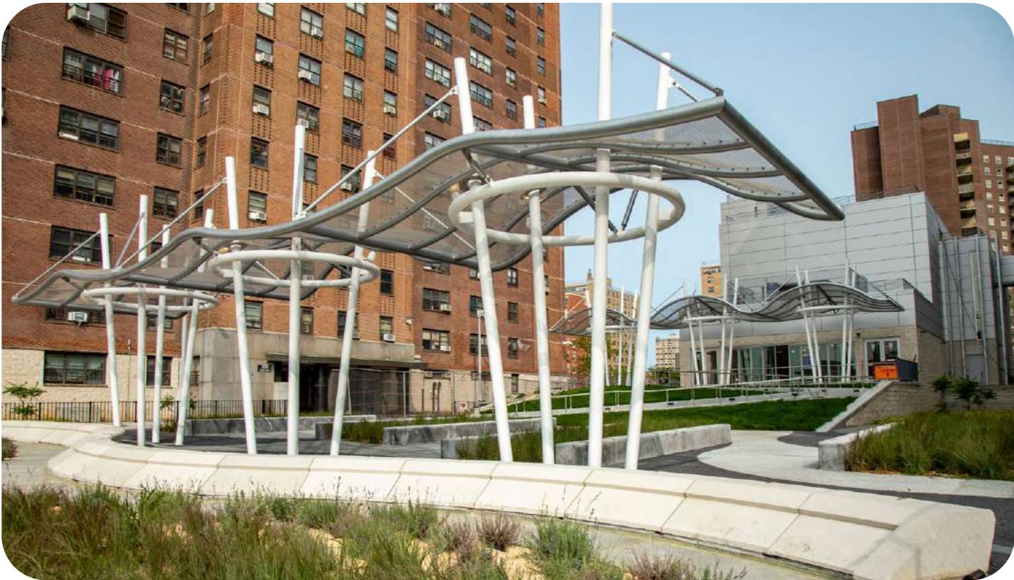
Community space created within and adjacent to the new boiler plant in Coney Island Houses
