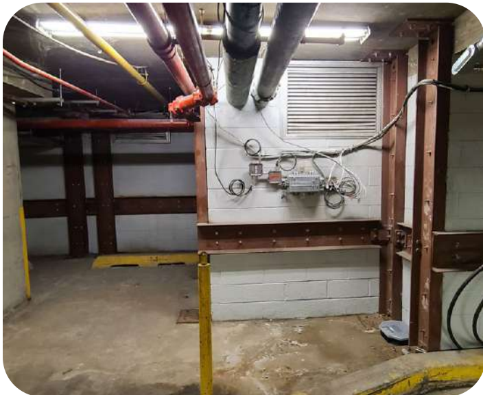
Two Bridges: Structural reinforcement inside the gas room and outside of the fire pump room
