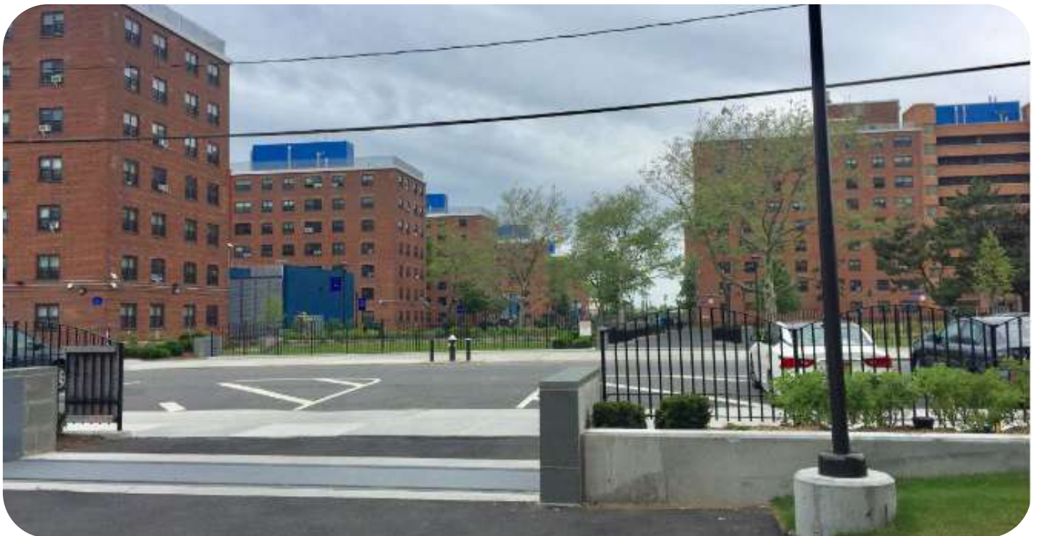
Passive flood gate and flood wall
