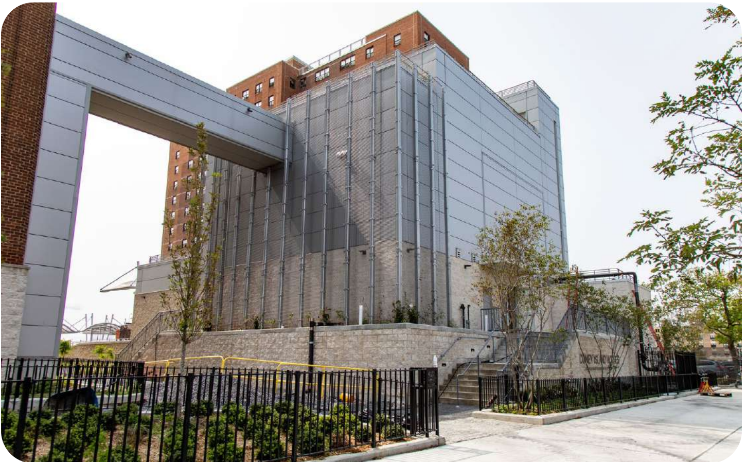
The new MEP annex at Coney Island Houses contributes to a renewed image of the development
