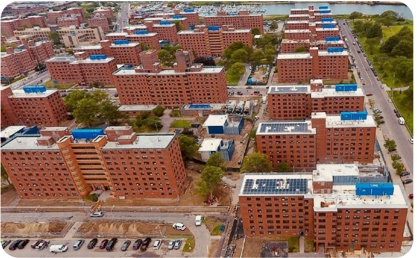
Rooftop hydronic boilers and elevated structures housing generators and electrical equipment
