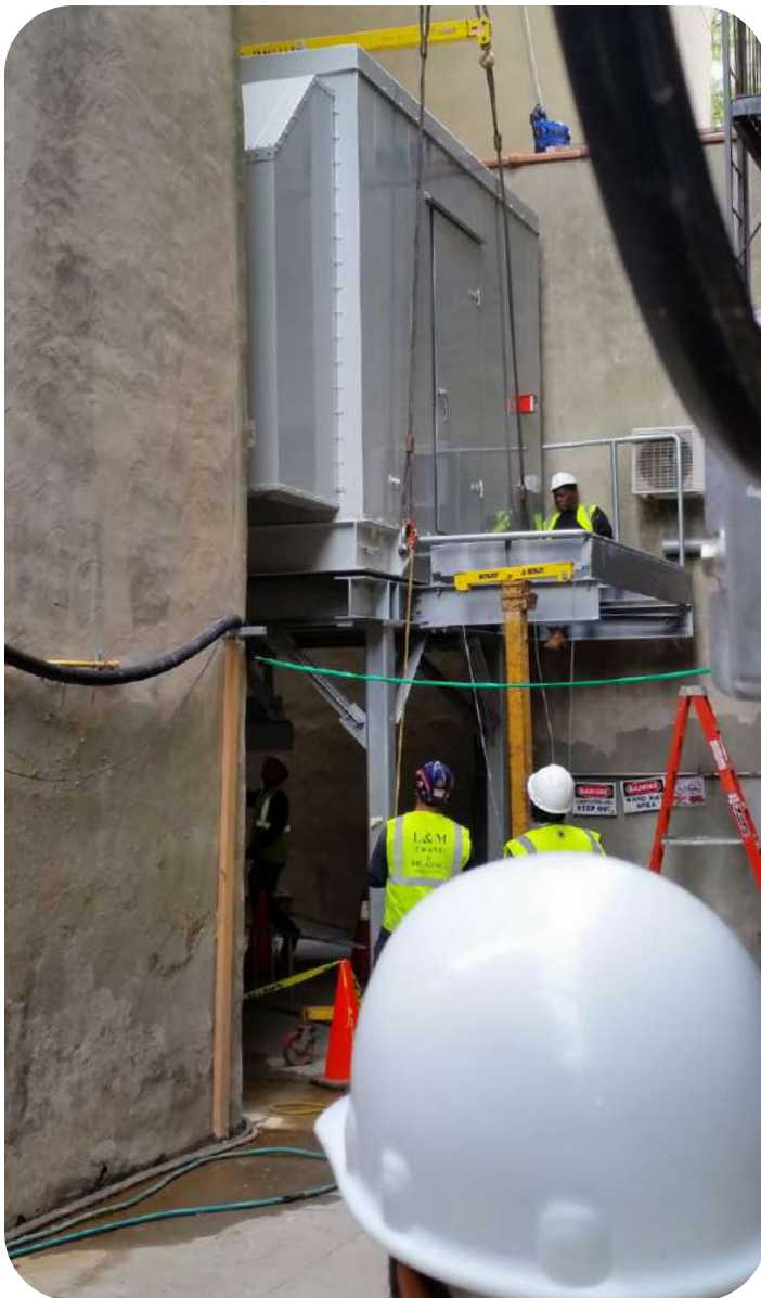
Installation of a generator on post at Lower East Side V
