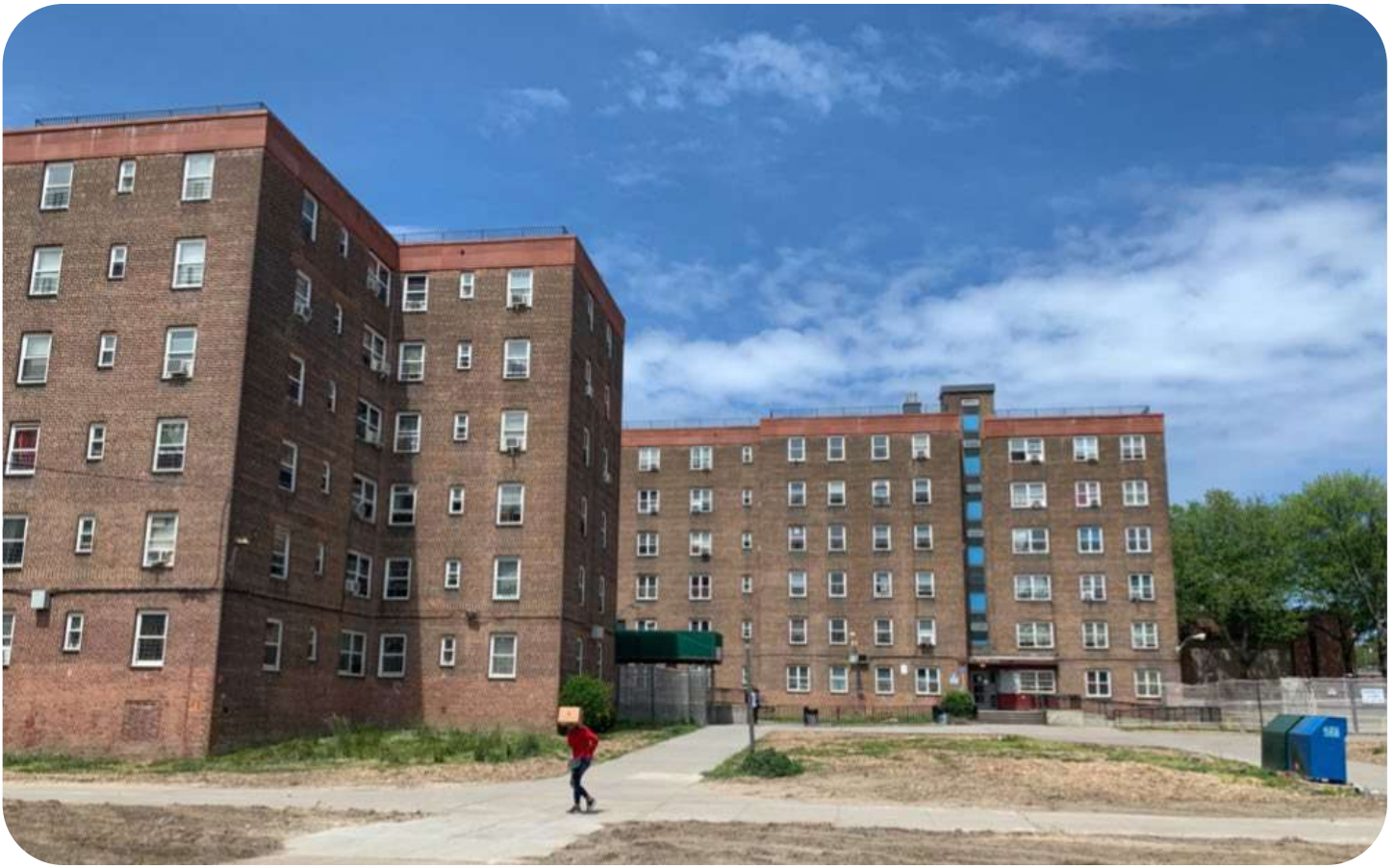
Red Hook green spaces in poor condition in May 2020
