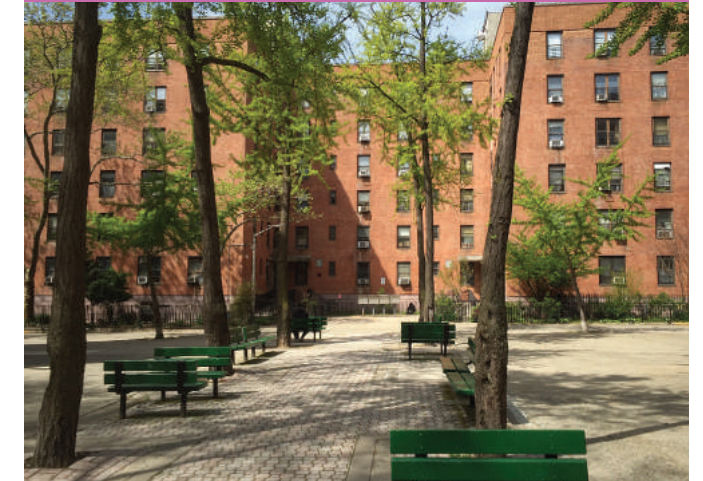
Red brick pavings at Vladeck Houses, where color differentiation of pathways highlights important areas of the campus.
